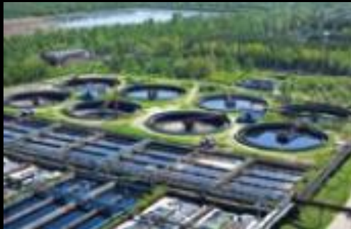
Waste & Waste Water
