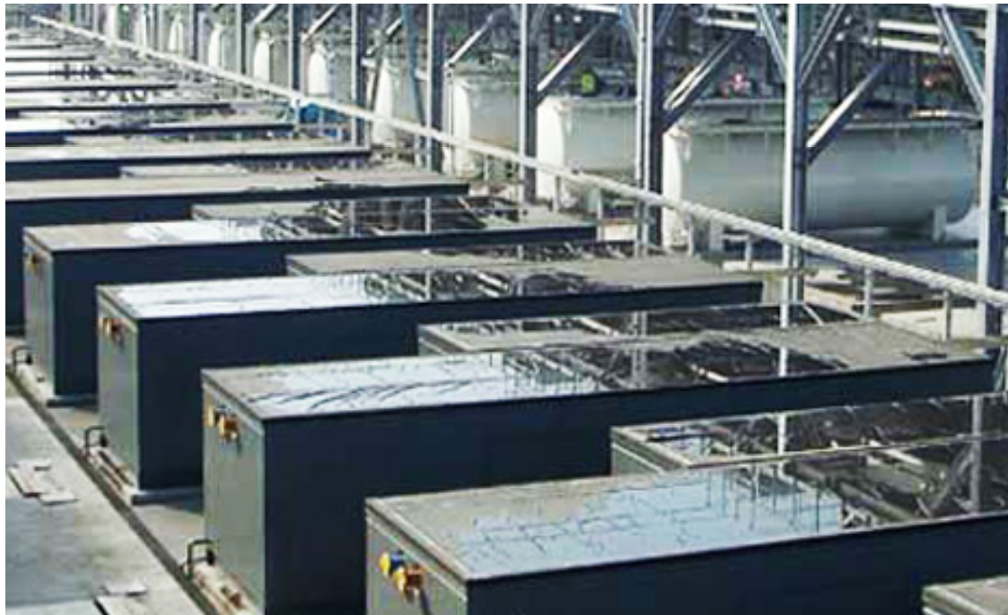
Google Data Center in Belgium
