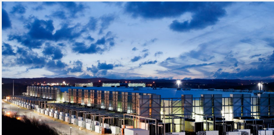
Douglas County, Georgia. Google Data Center. Photo: Google/Connie Zhou.
