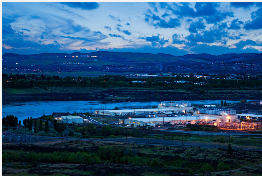
The Dalles, Oregon. Google Data Center. Photo: Google/Connie Zhou.
